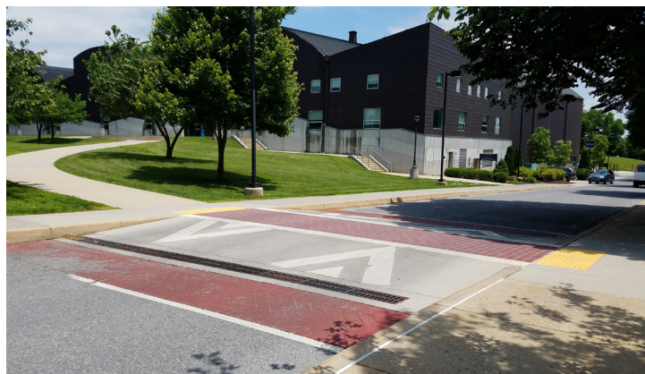
This is a raised crosswalk on a university campus. This crosswalk contains an in-road drainage system, which is not typically found at a speed table on municipal streets.
